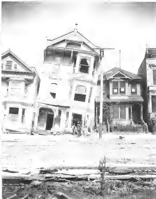
FIGURES 26–27. Figure 26 (left). Howard near 17th, San Francisco. Buckling of rails by compression. G.K. Gilbert photograph [GKG 2879], U.S. Geological Survey Photographic Archives, Denver, Colorado (also pl. 91 in Lawson [1908]). Figure 27 (right). Howard Street near 17th (East side of street). All houses shifted toward left. Tall house (center) dropped from its south foundation. G.K. Gilbert photograph [GKG 2893], U.S. Geological Survey Photographic Archives, Denver, Colorado.
